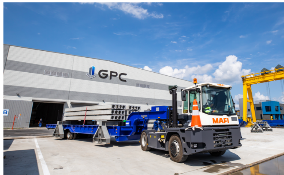
Precast Concrete (PC) plant in Eumseong-gun, Chungcheongbuk-do
