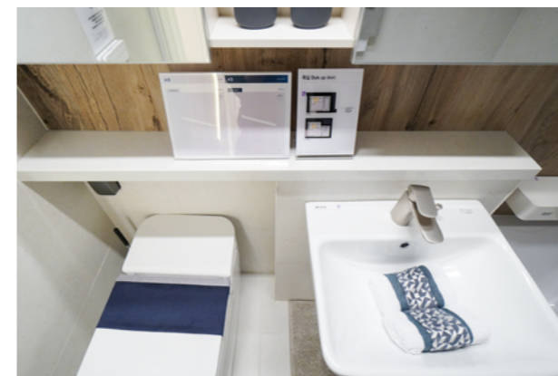
Bathroom Shelf Constructed with Engineered Stone
